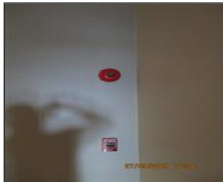
Photo of the dormitories (if applicable) Fire alarm has been installed at owner residence at 7th floor.jpg
