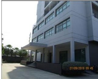
External photo(s) of the production unit(s) Factory building_4.jpg
