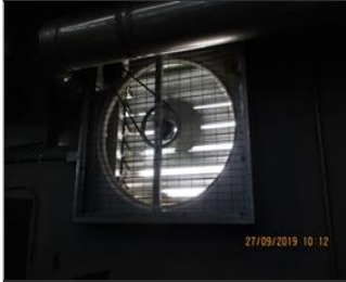
Photo of chemical storage room (if applicable) Ventilation fan.jpg
