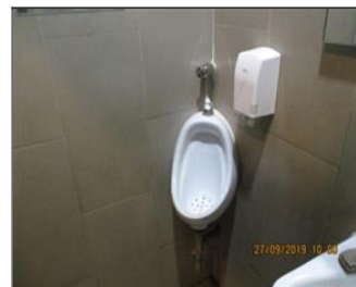
Photo of the sanitary facilities Male toilet_2.jpg
